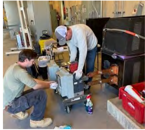
Contractors working on NTP's breakers
