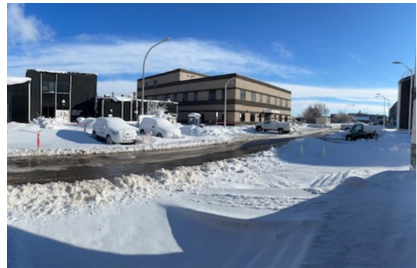
Main entrance to new OSCB
