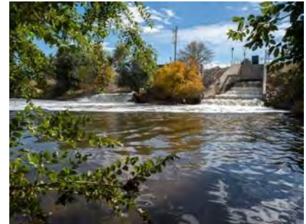
Outfall area at the RWHTF, where treated wastewater (effluent) is returned to the South Platte River
