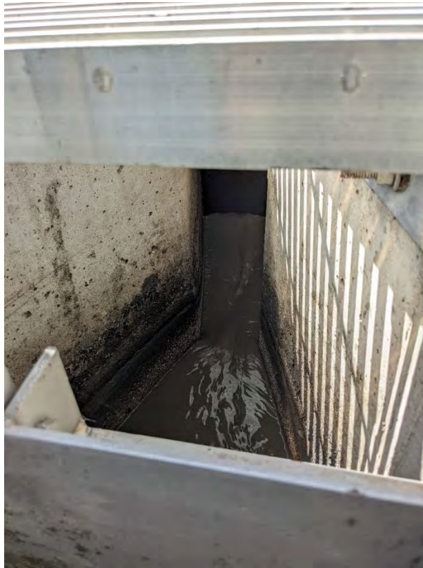
Fig. 2: WAS Flow into DAF Unit
