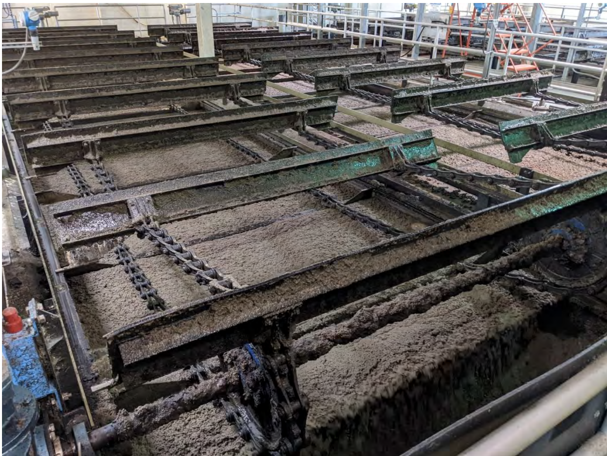
Fig. 3: CONWAS being skimmed off the DAF Unit
