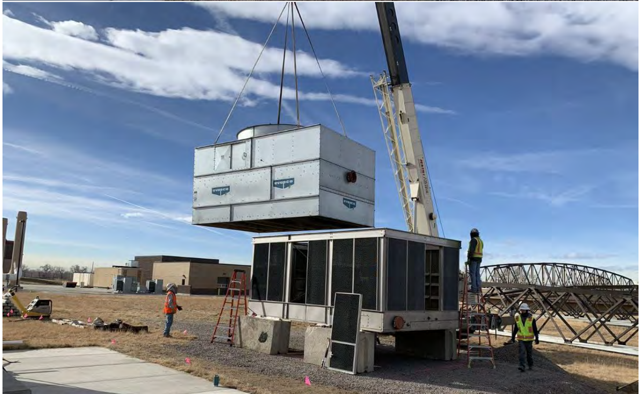
Delivery and Installation of Cooling Tower
