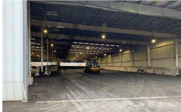
Approximately 20 loads in storage bay
