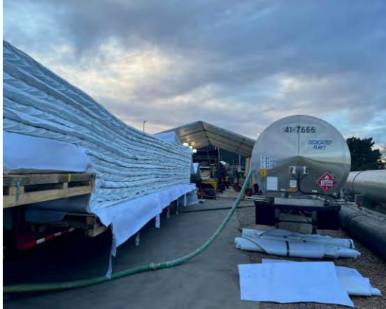
Cured in-place piping “sock”
