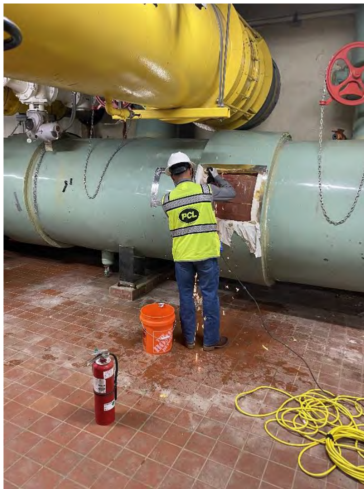
Figure 4 - Examining Aeration Header Couplings
