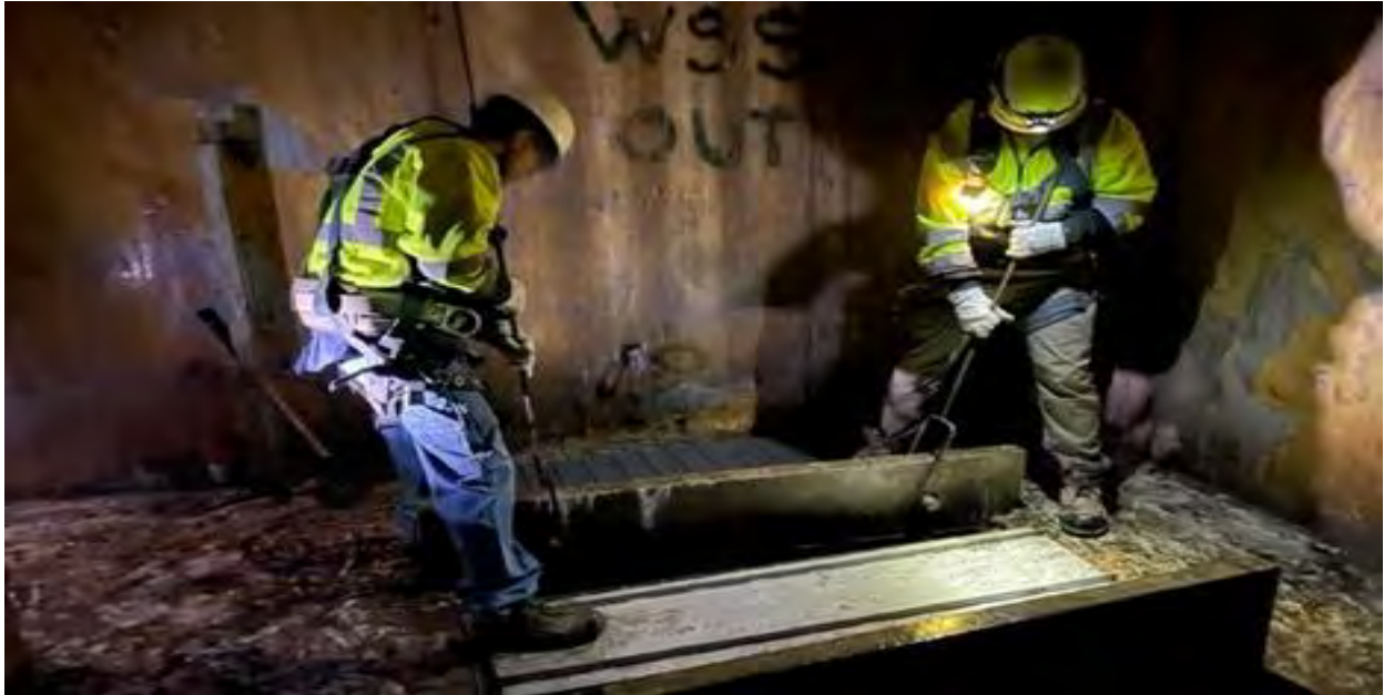
Transmission crew conducting a flow diversion.
