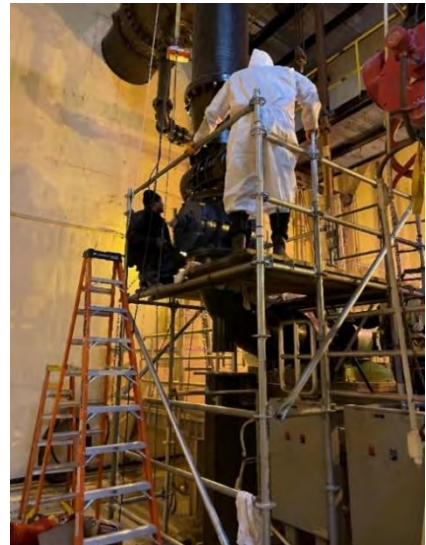
Scaffolding erected to reach valve.
