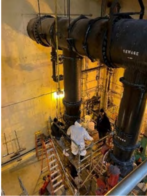
Mechanical crew replacing the valve at the lift station.
