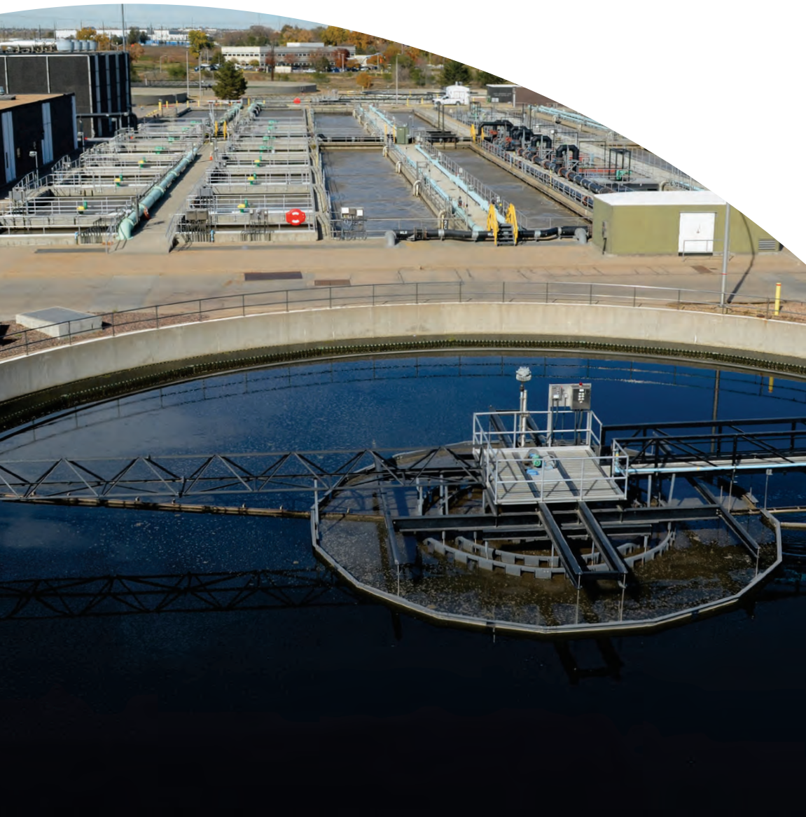
RWHTF North Plant clarifier and aeration basins.
