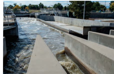
RWHTF influent channels.
