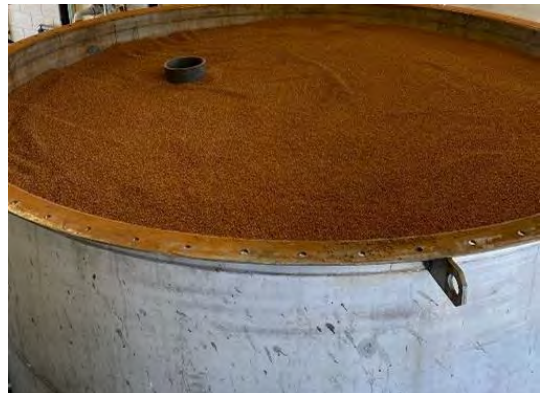
The tank is filled with new granular media.
