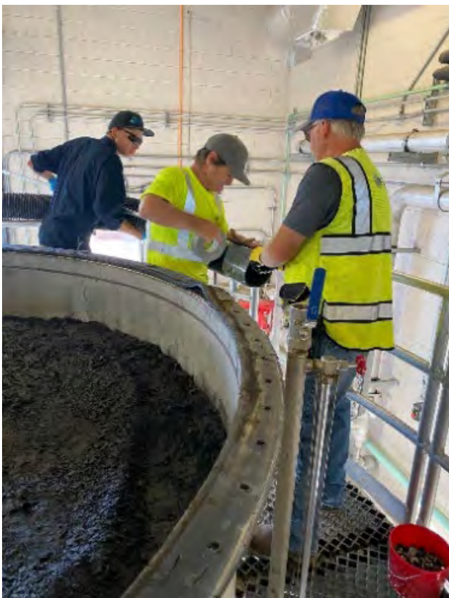
Top left: Earl Chappell and Jeremy Hileman working with contractor during iron sponge removal. Top right: Hydrovac discharging spent iron sponge media in NTP's lined pond. Center right: H 2 S removal vessel filled with new ferrous hydroxide media. Bottom right: Sulfur Solve test skid.
