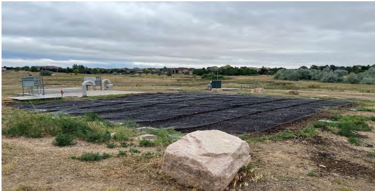
Complete filter replacement with wire netting.
