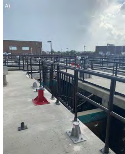
Safety improvements to the 630 Tertiary Flocculation/Sediment Basins, including new personal and equipment davits, access gates, and ladder stops.
