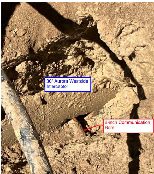
Figures 4 & 5: Lumen Bore in Metro Interceptor from Outside (Left) and Inside (Right) of the Pipe
