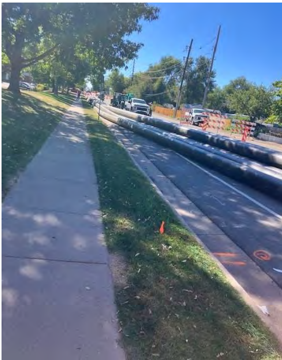
Pipe staging for first bypass (left) and temporary trench under intersection (right) near S. Dayton St. and S. Parker Rd.
