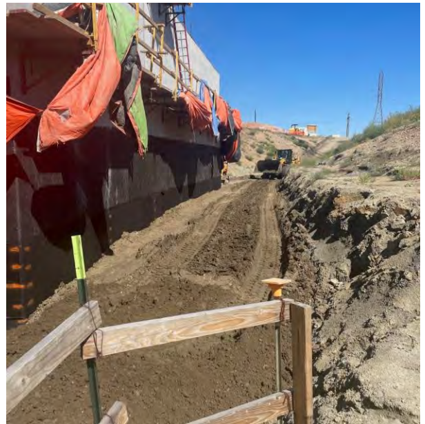
New lift station structure (left) and backfilling of south wall (right)
