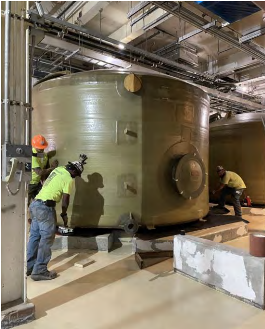
Placement of an emulsion polymer tank (left) and demolition of the DSSF (right)
