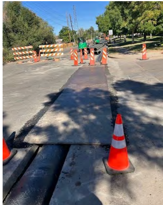
Pipe staging for first bypass (left) and temporary trench under intersection (right) near S. Dayton St. and S. Parker Rd.
