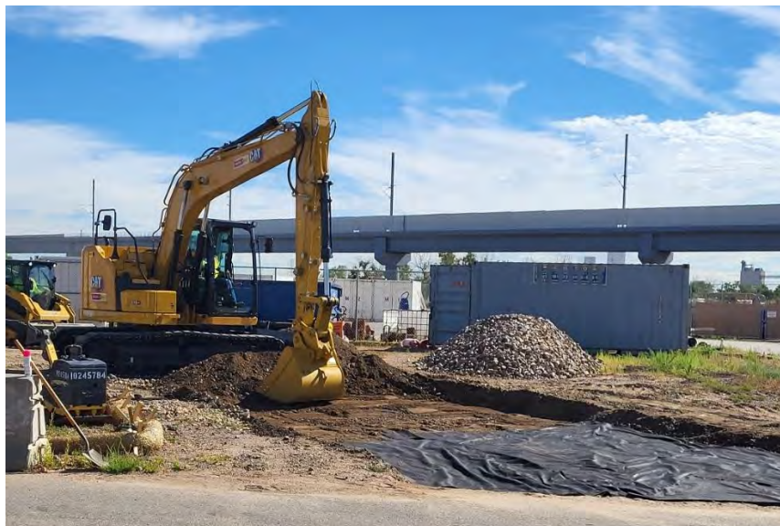
Constructing temporary access for South PAA chemical delivery
