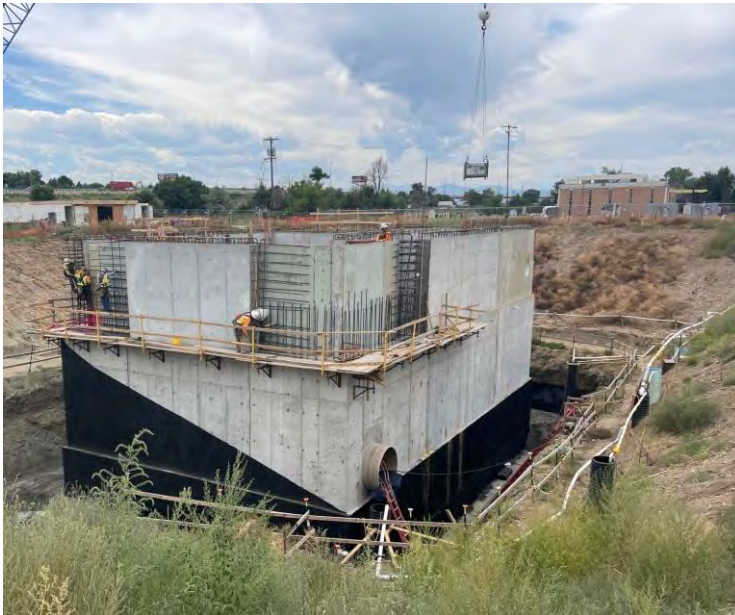
New lift station structure (left) and backfilling of south wall (right)
