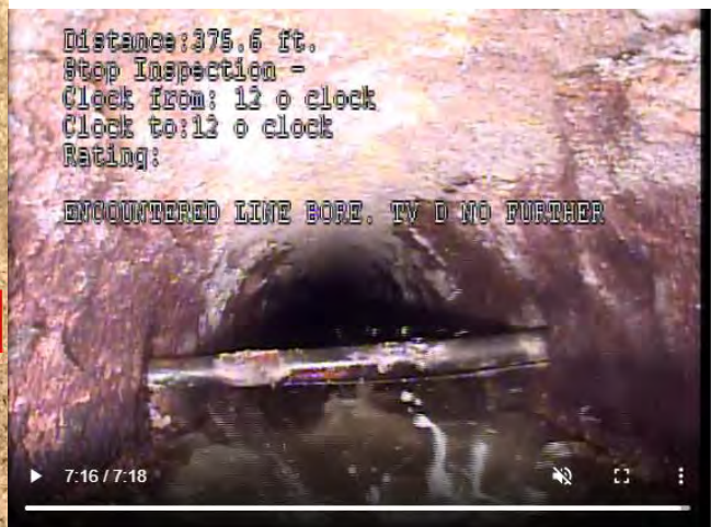
Figures 4 & 5: Lumen Bore in Metro Interceptor from Outside (Left) and Inside (Right) of the Pipe
