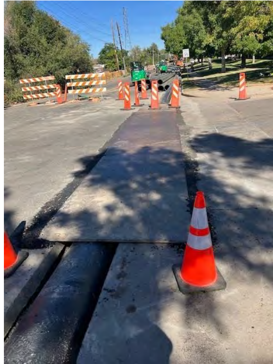
Figures 2 & 3: Pipe staging for first bypass (left) and temporary trench under intersection (right)
