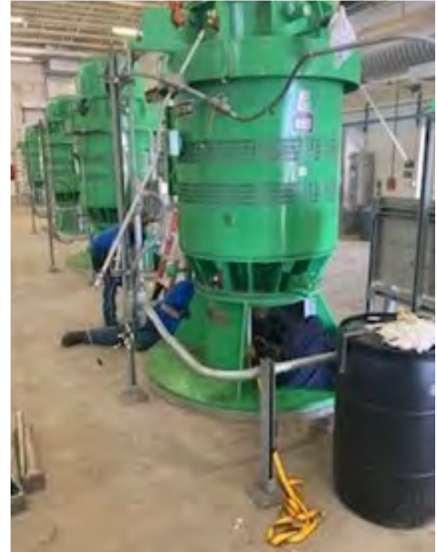
De-coupling the pump.
