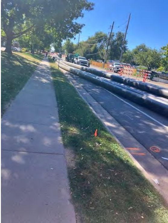
Figures 2 & 3: Pipe staging for first bypass (left) and temporary trench under intersection (right)
