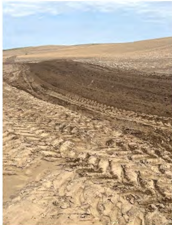
Filling washes with tractor and construction disc.
