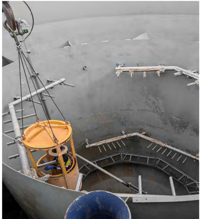
Man basket inside reactor.
