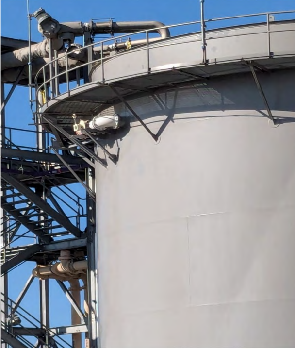
Second penetration (white pipe) for new effluent line.
